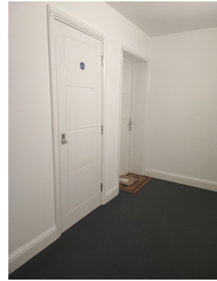
Example electrical riser.
